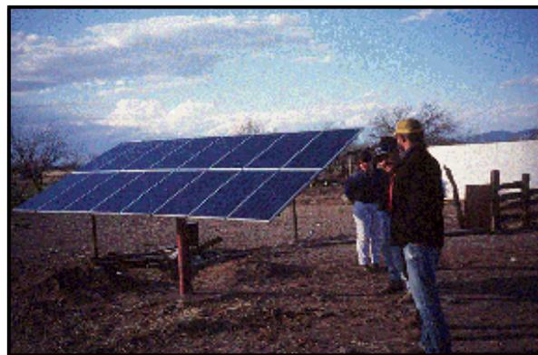
**Figure 1. Typical program installation: PV water pumper in Rancho Jeromin, Aldama, Chihuahua.**
